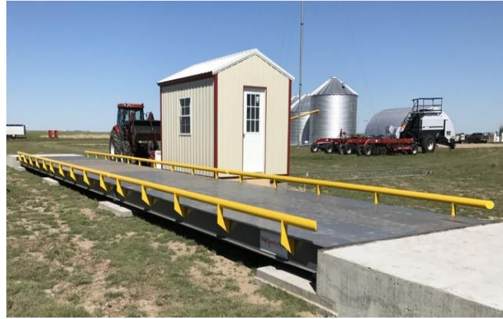
3" Weld-On Pipe Side Rails
